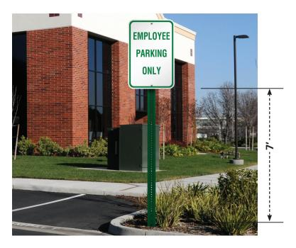
In urban areas, signs shall be installed a minimum of 7 feet (measured vertically from the bottom of a sign to the top of a curb or elevation of the near edge of the traveled way in the absence of a curb) in business, commercial, or residential areas at the side of the road where a pedestrian may traverse.
